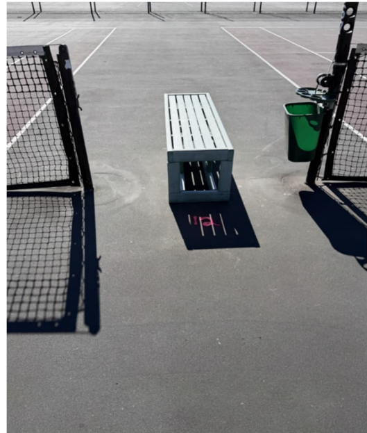
Photo 4: Small cracking at net poles at DCP-12
